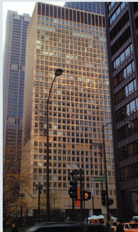
Exterior view of 69 West Washington
