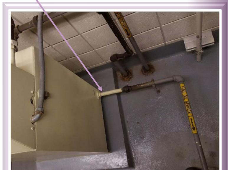
**Figure 2:** 50-gallons day tank with no shutoff valve and bottom connection incorrectly below the liquid level of the tank.
