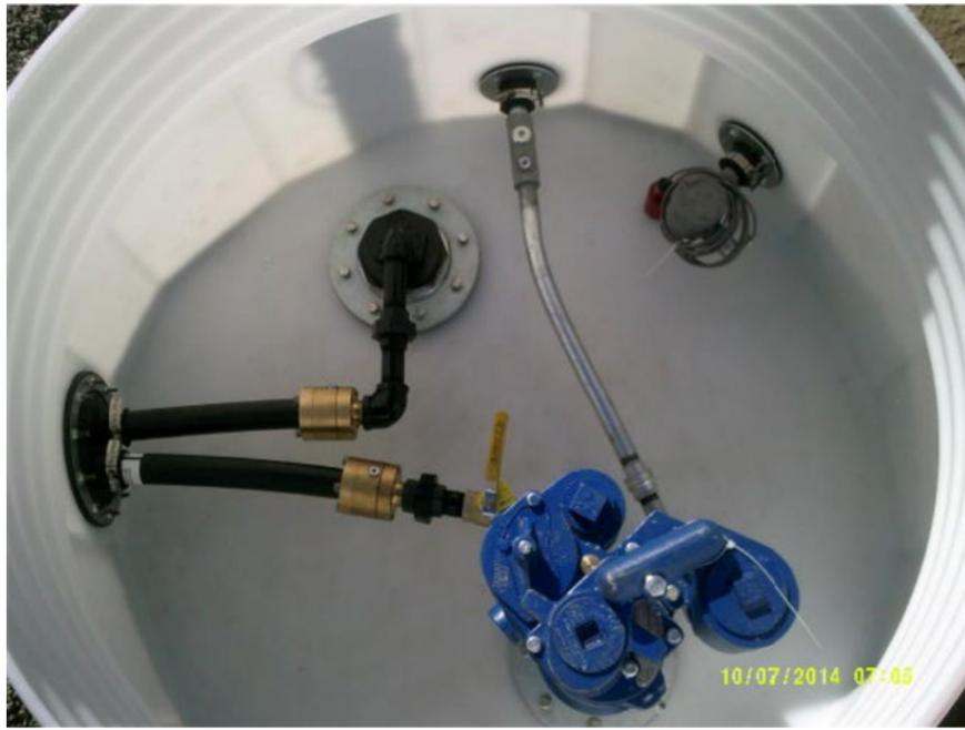
*Figure 14: Sump containing submersible pump head, pressurized supply piping and a return pipe.*
