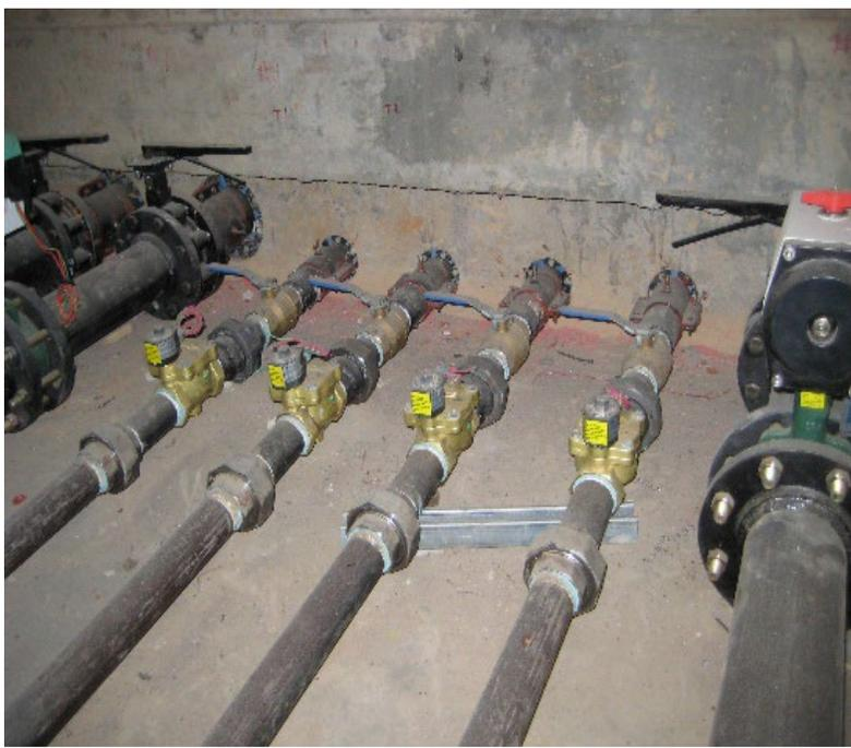
*Figure 9: Illustration of aboveground piping above floor of basement. This section of piping is exempt from federal UST technical prevention requirements but may be subject to the SPCC regulation. Note that the section of the piping back to the underground tank (not shown) that is routed through the concrete, but most importantly is in contact with soil, must meet federal UST release detection requirements.*
