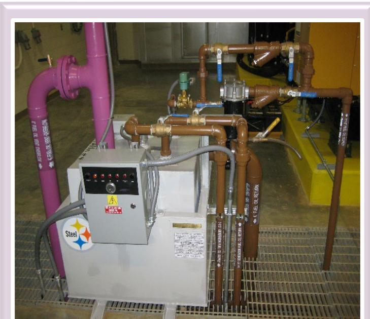
*Figure 10: Illustration of piping in trenches covered by see-through metal grating.*
