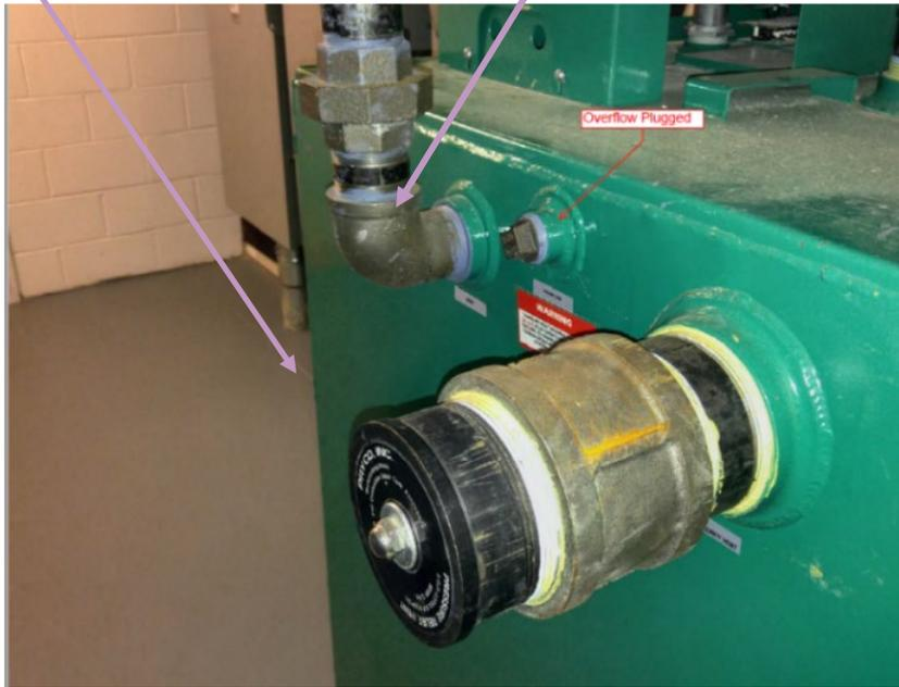
**Figure 5:** 400-gallons day tank with plugged overflow and emergency vent below liquid level.
