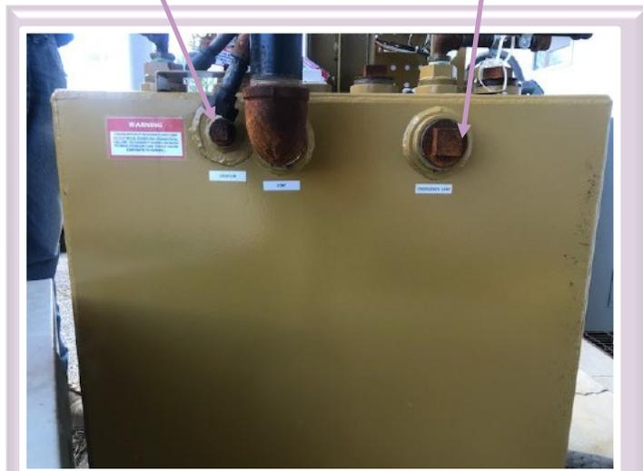
**Figure 3:** 50-gallon day tank showing overflow and emergency vent plugged.
