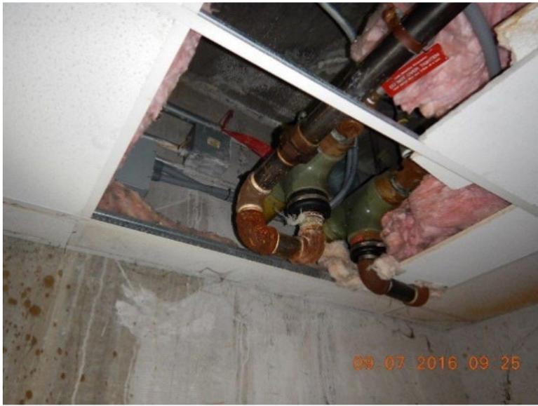
*Figure 8: Illustration of aboveground piping in a ceiling (here ceiling tile moved to expose piping) that is exempt from federal UST technical prevention requirements.*
