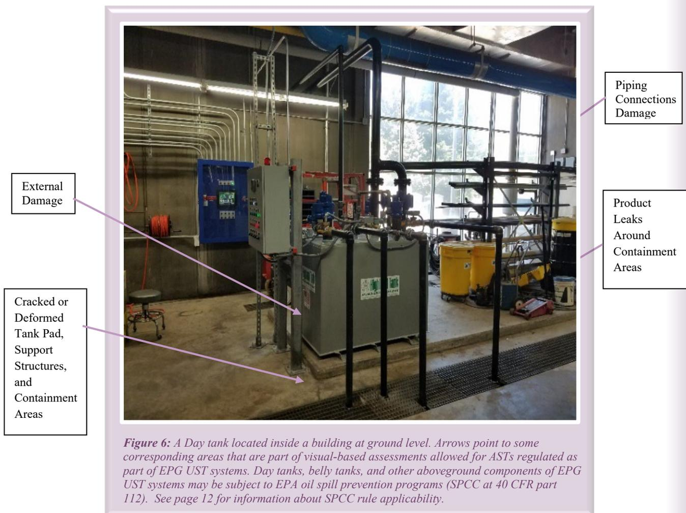
*Figure 6: A Day tank located inside a building at ground level. Arrows point to some corresponding areas that are part of visual-based assessments allowed for ASTs regulated as part of EPG UST systems. Day tanks, belly tanks, and other aboveground components of EPG UST systems may be subject to EPA oil spill prevention programs (SPCC at 40 CFR part 112). See page 12 for information about SPCC rule applicability.*
